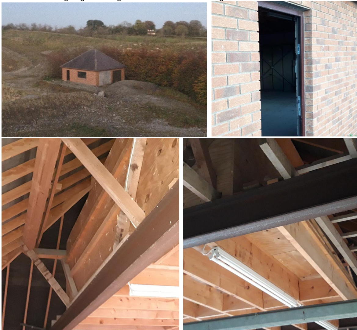
Plate 2: Disused garage showing internal structure of building
