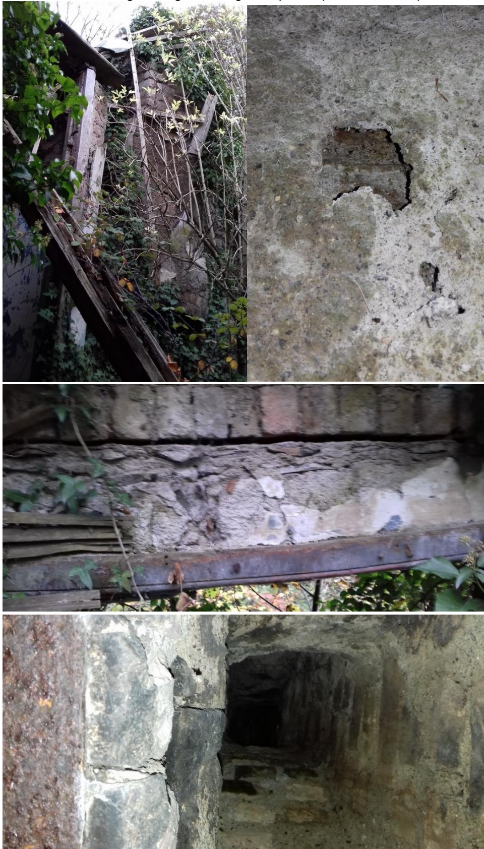
Plate 1: Abandoned gate lodge showing examples of potential roost spaces
