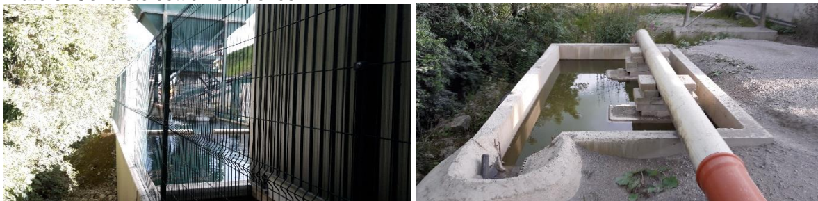
Plate 3: Concrete settlement ponds
