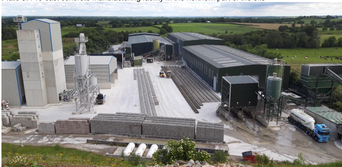
Plate 9: Pre-cast concrete manufacturing facility in the northern part of the site
